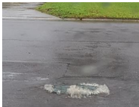
Overflowing sewage at 42 nd Ave. S at 41 st St. S
